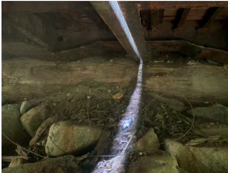
Right Bank Abutment when facing downstream
