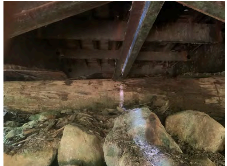
Left Bank Abutment when facing downstream
