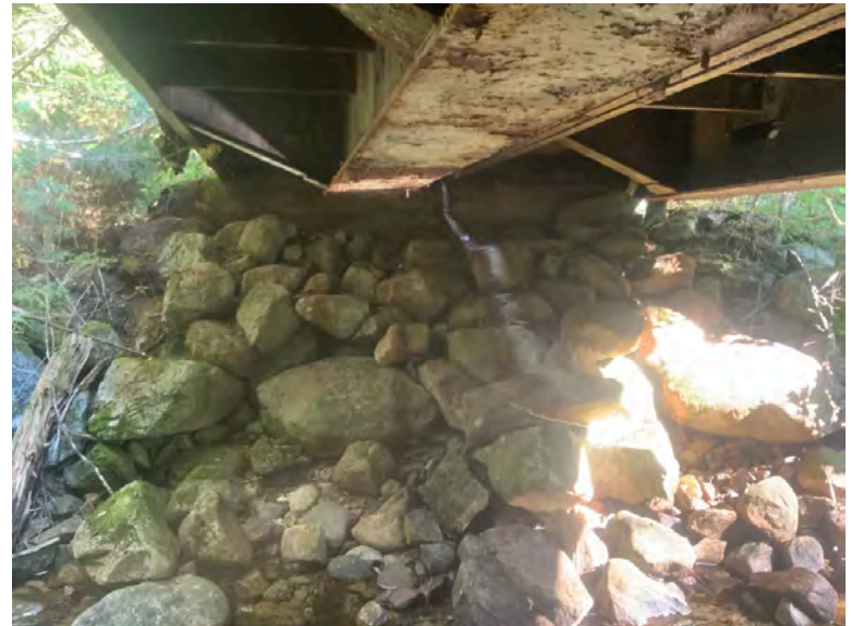
Right Bank Abutment when facing downstream
