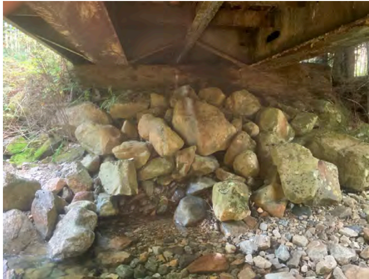
Left Bank Abutment when facing downstream
